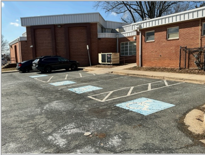
OVERVIEW OF ACCESSIBLE PARKING AREA
