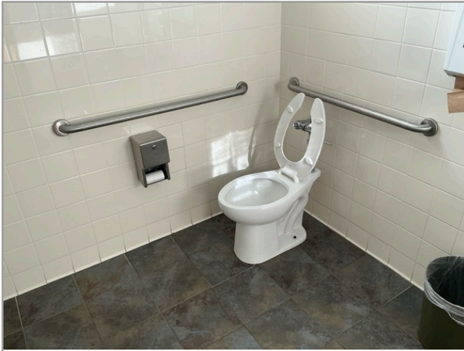
TOILET STALL OVERVIEW
